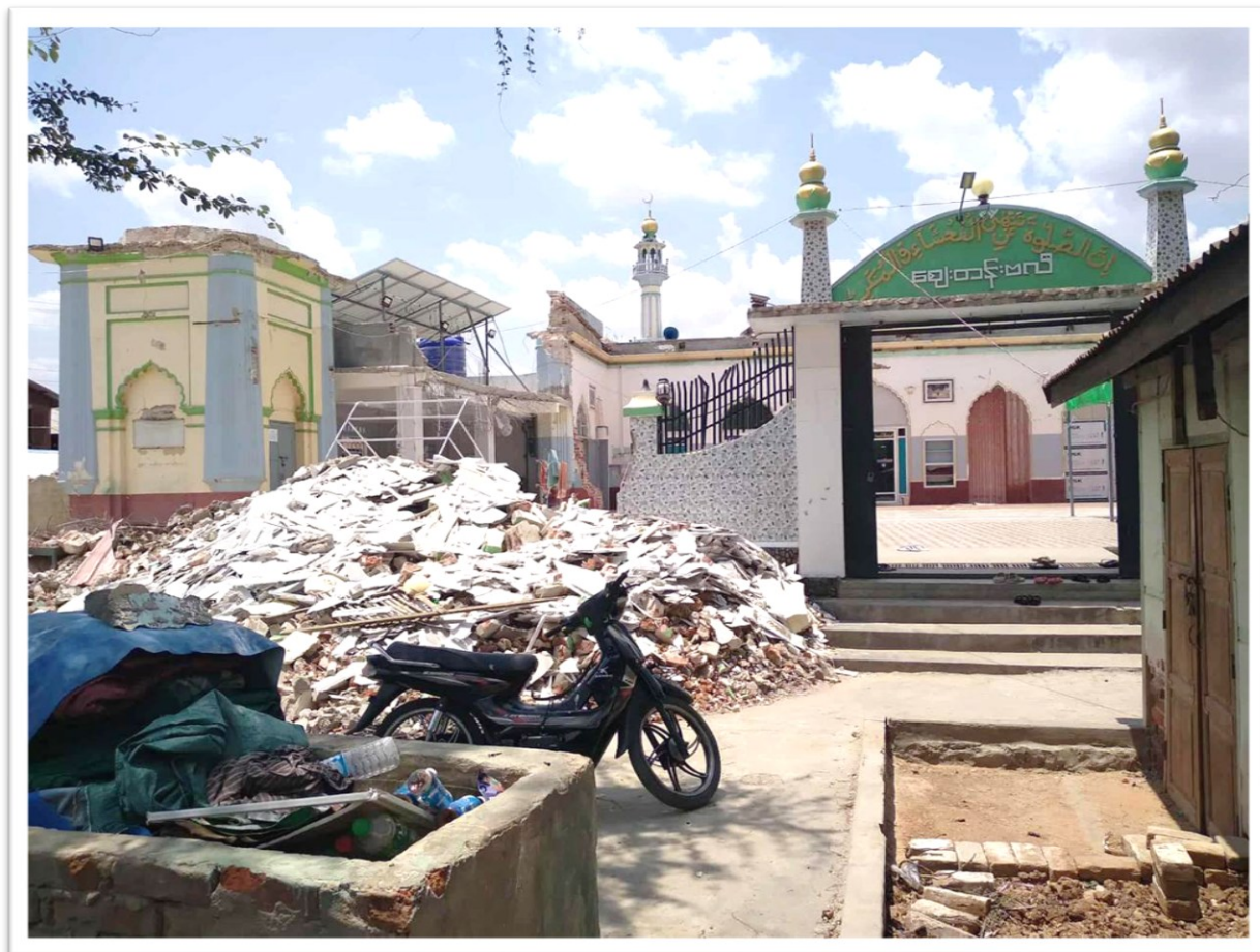
The Zay Tan Mosque in Yindaw Ywama village, Pyawbwe Township, Mandalay Region, after collapsing in the March 2025 earthquake. © BHRN, 2025.
