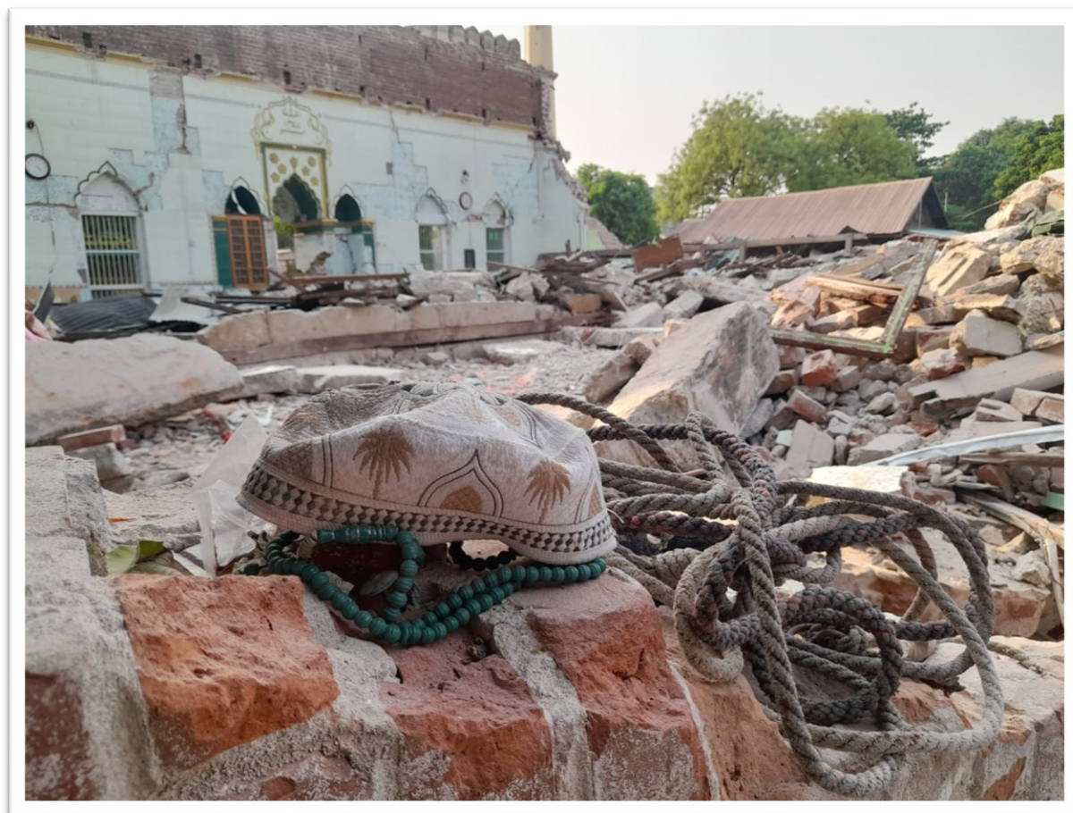
The Myoma Mosque in Sagaing Township after the 2025 earthquake. © BHRN, 2025.
